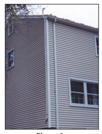
**Figure 9**Vent Line Installation (2 inch)
